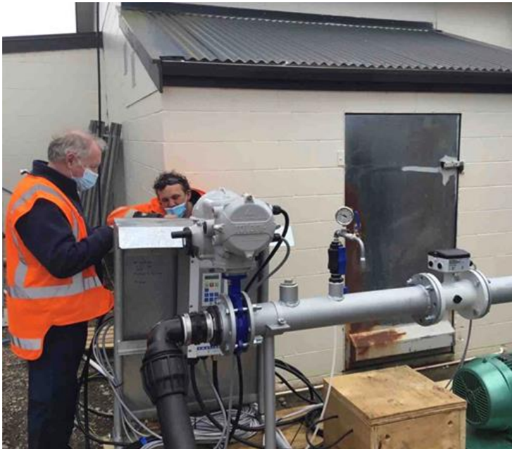
Figure 4. Commissioning works at Waiohine WTP
