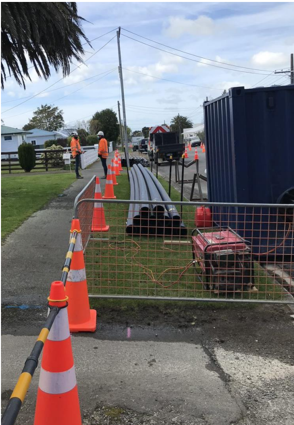
Figure 7. Site works on Fox St water main, Featherston
