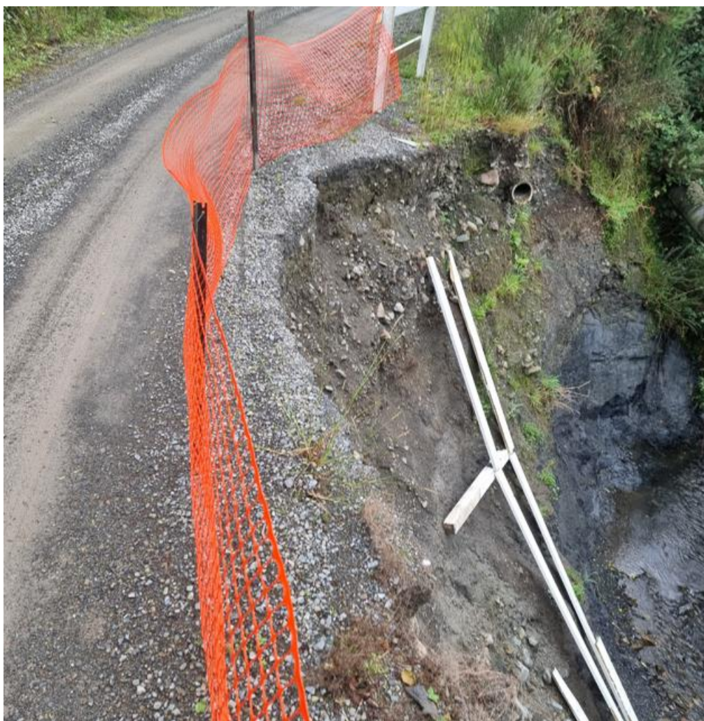
Figure 4. Boar Bush Gully Road slip, April 2022
