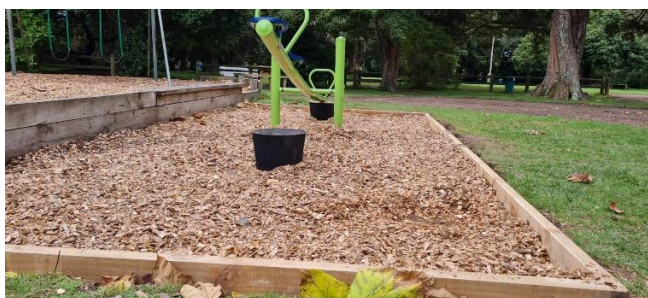
Figure 2. Greytown Playground seesaw replacement
