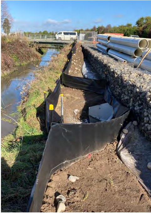
Figure 6 Sediment controls and gabion baskets next to Tilsons Creek
