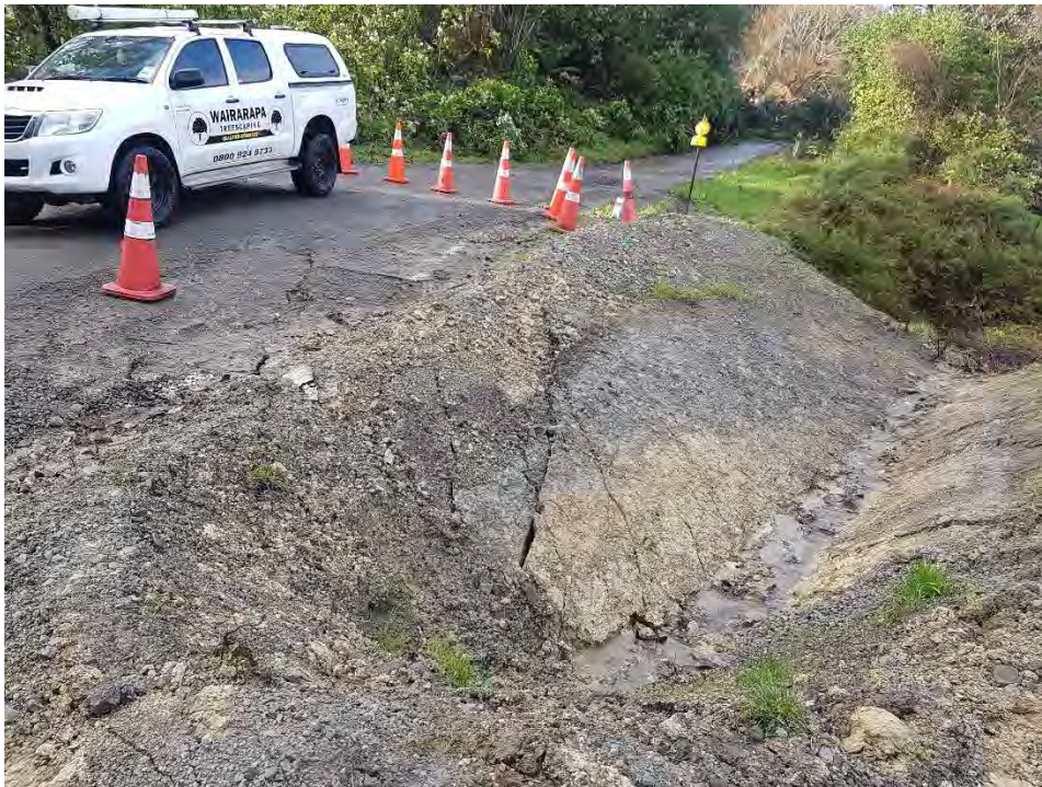
Sharp tension cracks in (1 year old) drain
