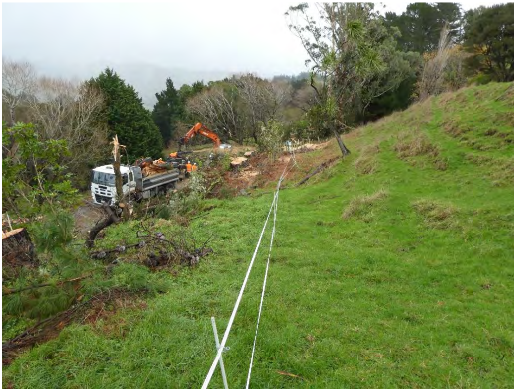
Lower slope above road landslide has pushed and tilted pine trees at top of steep slope above road (which have been cut down this week to the right – photo below)
