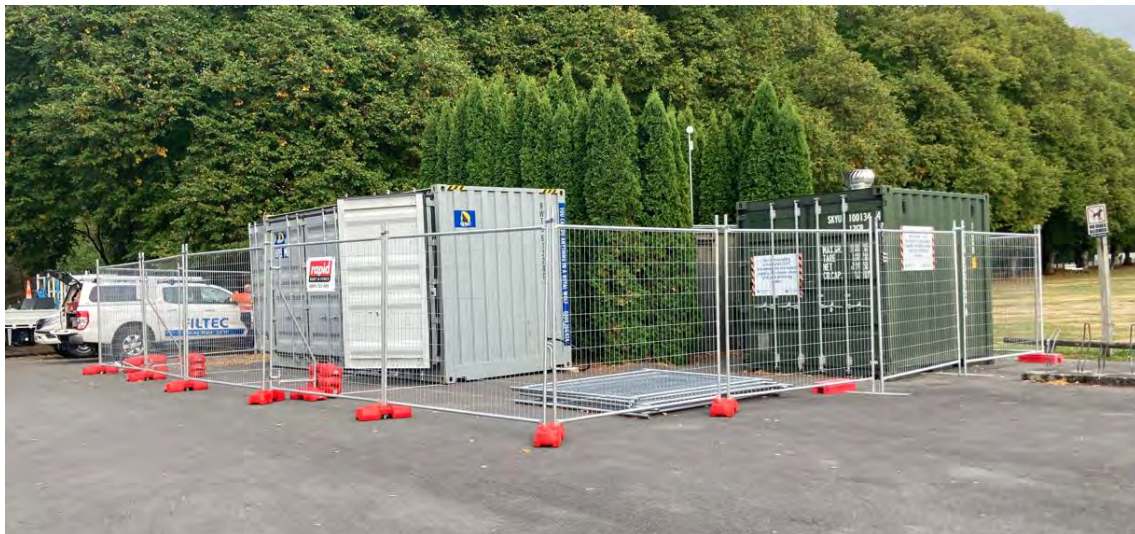
Figure 5 Temporary pH correction and UV treatment at Memorial Park bore
