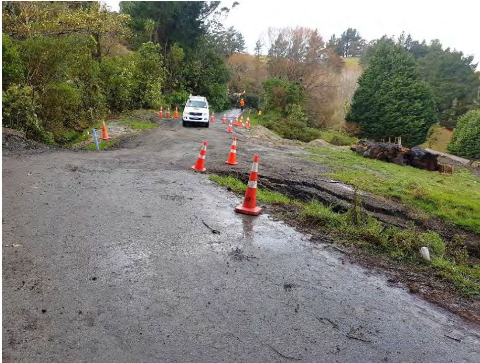
Approx. 4-5m offset of original white edge line to right of cones
