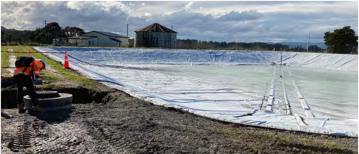
Figure 3 Final touches to the outlet pipe before commissioning starts on the treated water reservoir bladder (white)
