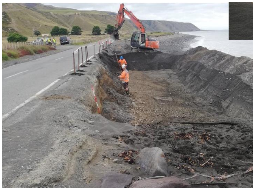
Excavation in preparation of ECOREEF installation
