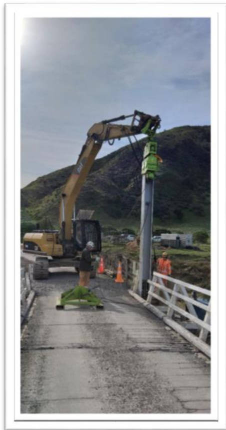
Pile driving Tora farm Settlement bridge.
