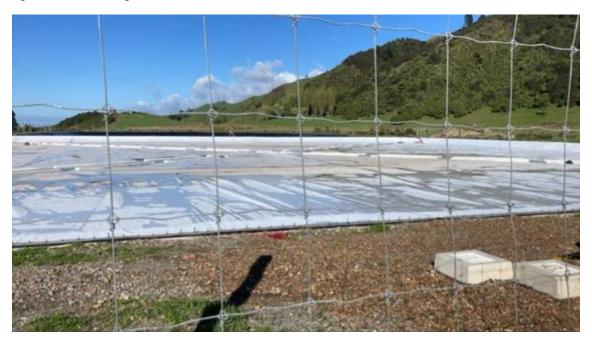
Figure 5. Photo of filled treated water reservoir bladder at Waiohine WTP
