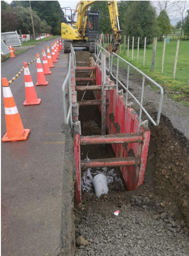
Figure 6. Photo of trenching works on Pah Rd, Papawai
