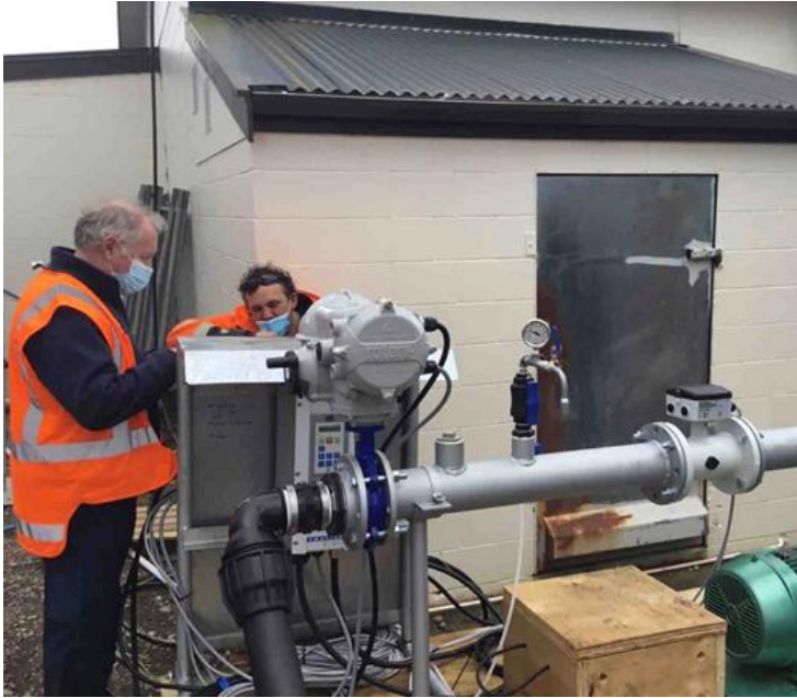
Figure 4. Commissioning works at Waiohine WTP
