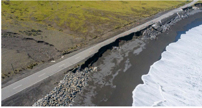
Coastal damage before.
