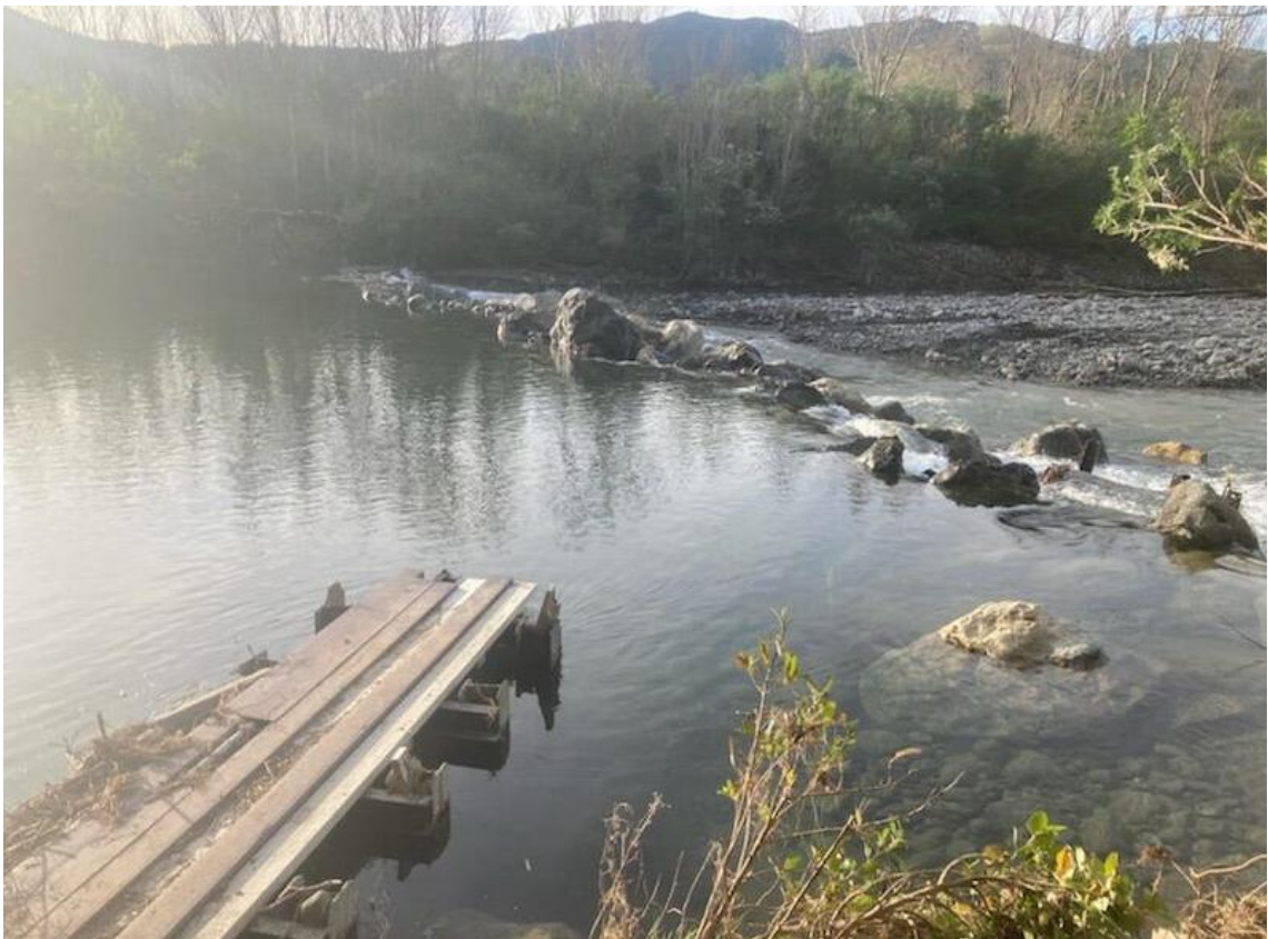
Figure 3 Longwood race intake rock weir being reinstated
