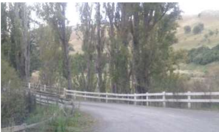
Figure 6.3b Bridge, Ruakokopotuna required structural assessment
