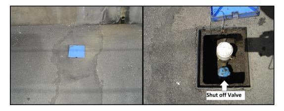
If required the water supply to your house can be turned off by turning the shut off valve shown clockwise
