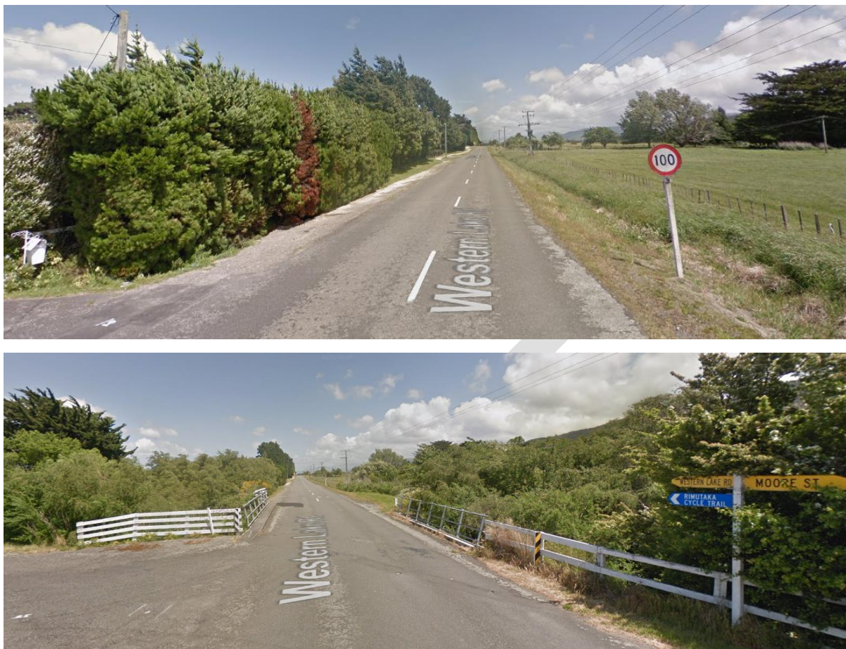
Figure 3.2: Existing location of speed limit threshold (up) and new location of speed limit threshold (down) looking south (Source: Google Maps)
