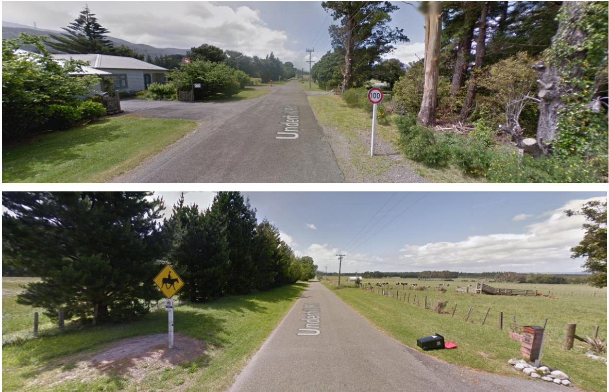
Figure 3.1: Existing location of speed limit threshold (up) and new location of speed limit threshold (down) looking north (Source: Google Maps)
