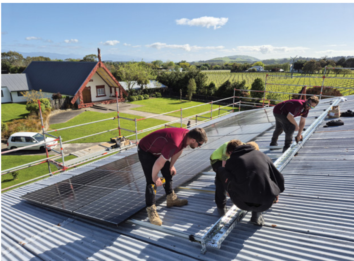
Hau Ariki Marae solar panel installation
