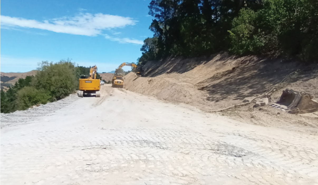
Hinekura Road remediation
