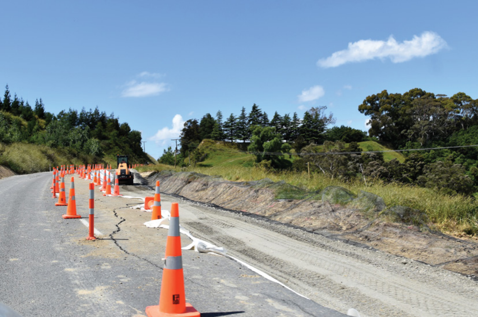
Ponatahi Road, Martinborough
