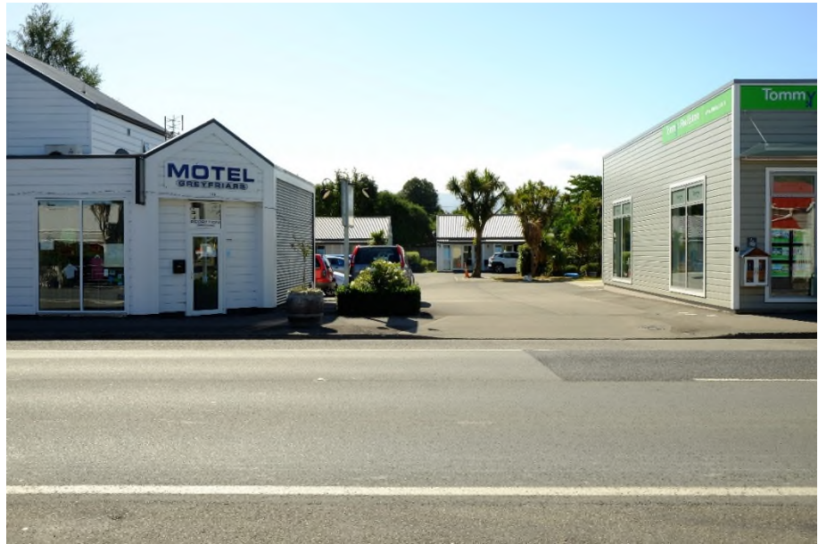
Figure 5: 10.5m wide gap at entrance to Greyfriars Motel, opening to wide area of parking, without enclosure provided by the large Beech Tree to be retained at the application site, not reducing in width into the site and without the further enclosure provided by planting along each side as proposed as part of the application.
