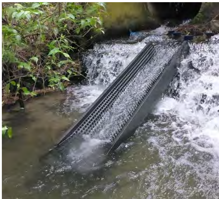
Figure 3.12: An example of a ramp to provide fish passage that could be installed on the weir to the residual flow.
