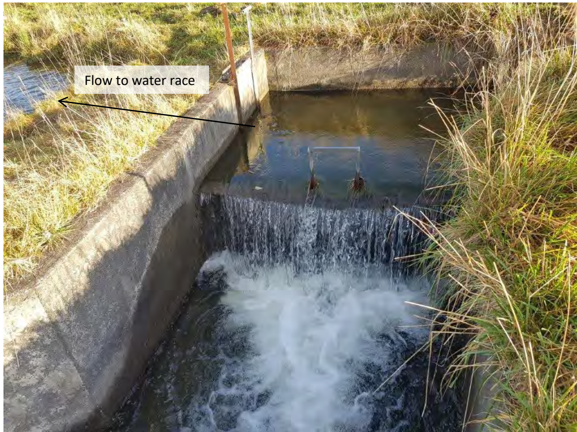
Figure 3.4: Longwood water race flow control structure showing the weir controlling the residual flow; the flow to the Water Race is via a culvert on the upper left of the picture, 3 June 2020.
