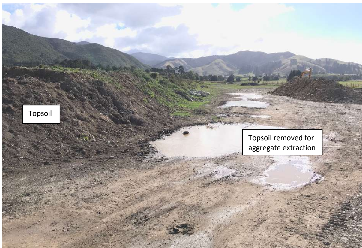
Photograph 1 - Topsoil stripped and aggregate ready for extraction to a depth of up to 4m
