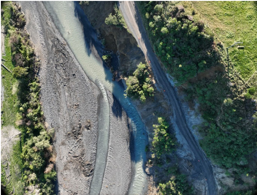
Figure 2: Landslide on both upslope and downslope at Whakatomotomo Road RP 2.650 to RP 2.850 (Drone image taken 02/07/2026)
