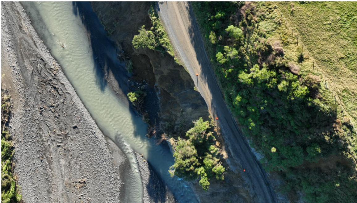
Figure 10: Toe of the underslip undermined by river scour (drone imagery captured on 2 July 2026)
