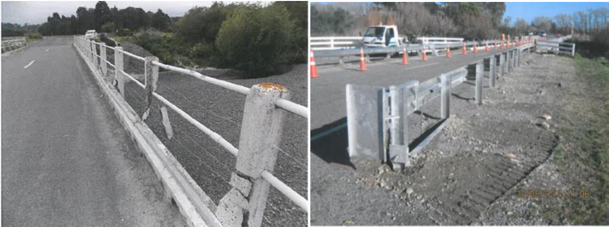
Figure 31 Bridge before and after prudential maintenance
